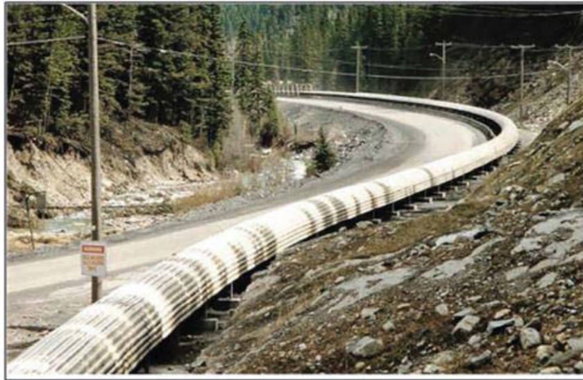
Figura 2-6. Sistema Metso Rope Conveyor Cable Belt.
