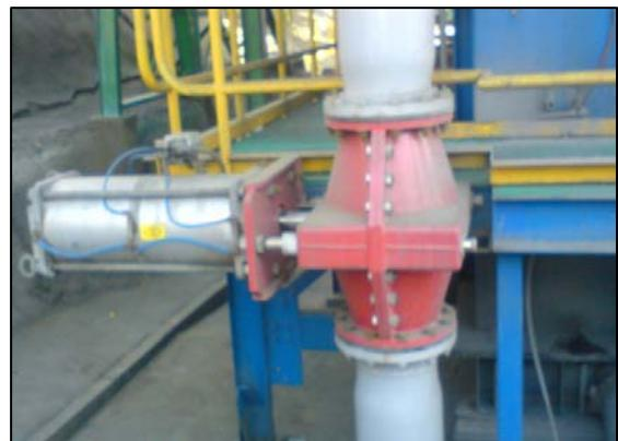
Figura 28: Válvula pinch.
