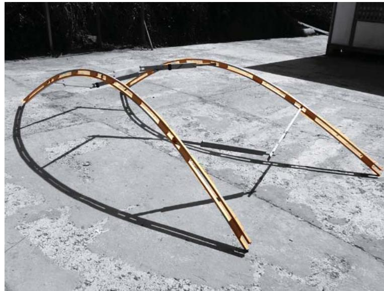
SE MUESTRAN LOS ARCOS CENTRALES LA BASE DE LA CUBIERTA, 2 VIGAS BASES.
