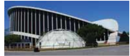
Raleigh Livestock Arena , North Carolina, 1952.
