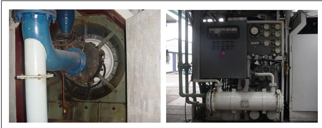
Figura 2.9 Compresor Booster C.02/C.03
