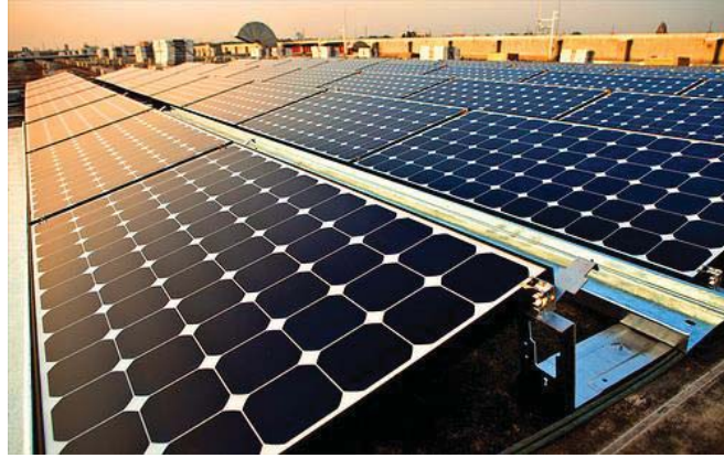
Figura 3-2: Paneles solares. (fuente: https://cdpmexico.wordpress.com )
